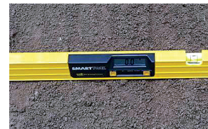
Laser control helps maintain the perfect grade
